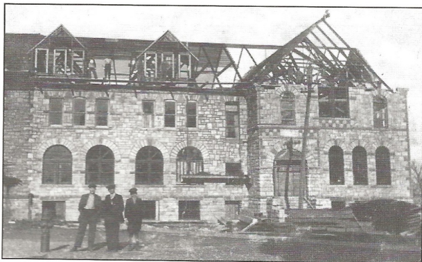
The school building during construction.
