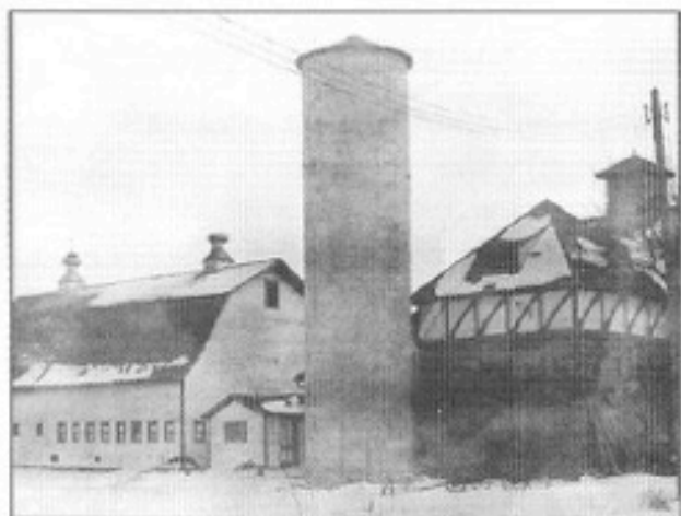
The first concrete silo in South Dakota.
