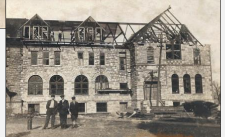
The Olde School expansion nearing completion in 1912, illustrating finished quartzite masonry alongside exposed roof framing prior to final construction.
